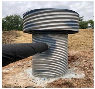
Riser replaced at Sediment basin 5 at Cell 6 North facing slope base.
