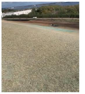
QRL cell 6 area (upper E slope) graded and hydro-seeded for soil stabilization as per MDE compliance requirement.
